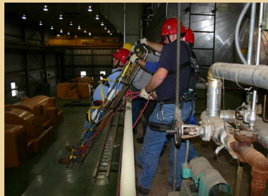
Parker and Guthrie help lower their patient to Plant Moselle's generator floor.
