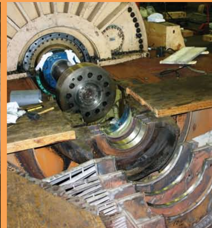
- Photos (top left) After being returned from Atlanta for repairs, the turbine rotor was carefully lifted to the turbine floor.
