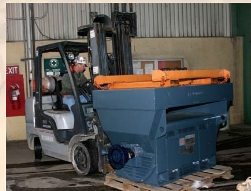
Mechanic I Landell Smith transports a primary air fan motor to be installed
