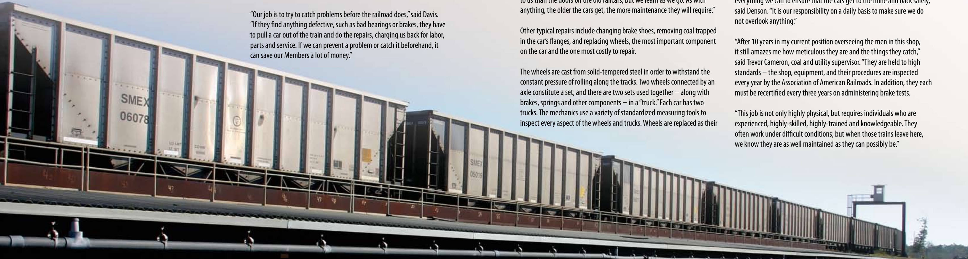
Coal trains at Plant Morrow can normally be unloaded in less than one hour
