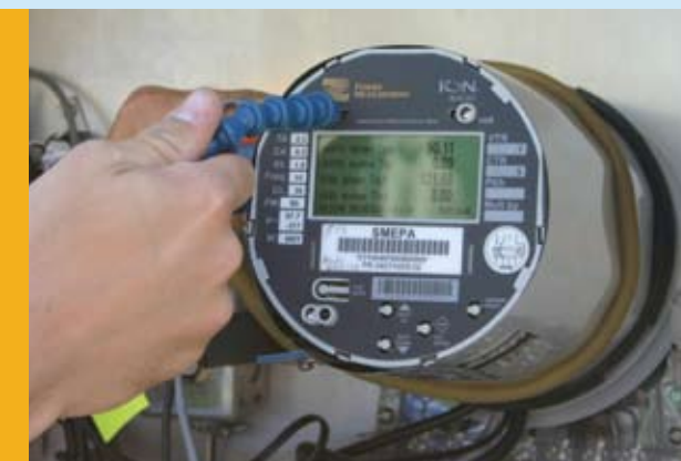
Lead Technician Jody Lott (far left) and Meter Technician Charles Hennis take readings at the Rawls Springs substation. SME has 185 metering locations throughout its on- and off-system. Each meter is capable of providing real-time data about voltage and current levels flowing from the transmission side of a substation to the distribution side. The data, which is regularly checked and verified, is accessible by computer for billing and testing.
