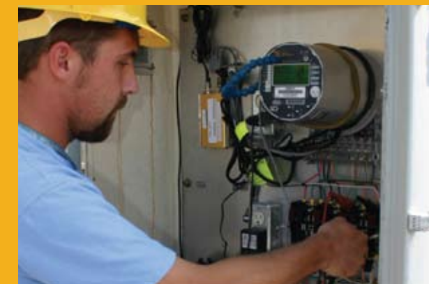
Lead Technician Jody Lott (far left) and Meter Technician Charles Hennis take readings at the Rawls Springs substation. SME has 185 metering locations throughout its on- and off-system. Each meter is capable of providing real-time data about voltage and current levels flowing from the transmission side of a substation to the distribution side. The data, which is regularly checked and verified, is accessible by computer for billing and testing.
